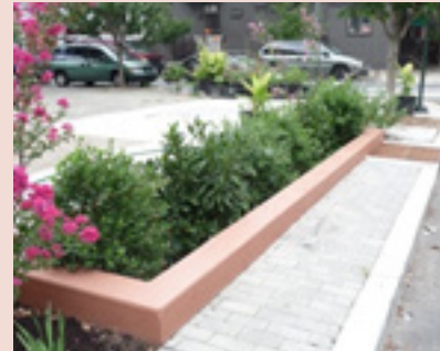
Stormwater planters designed for Columbus Square in Philadelphia.
