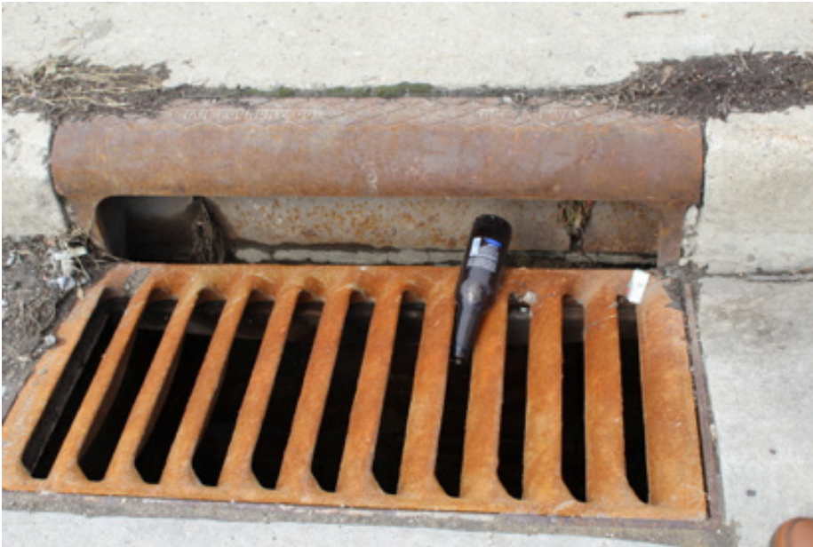
Figure 9: Trash in Storm Grate - Photo Courtesy of Luan Nguyen
