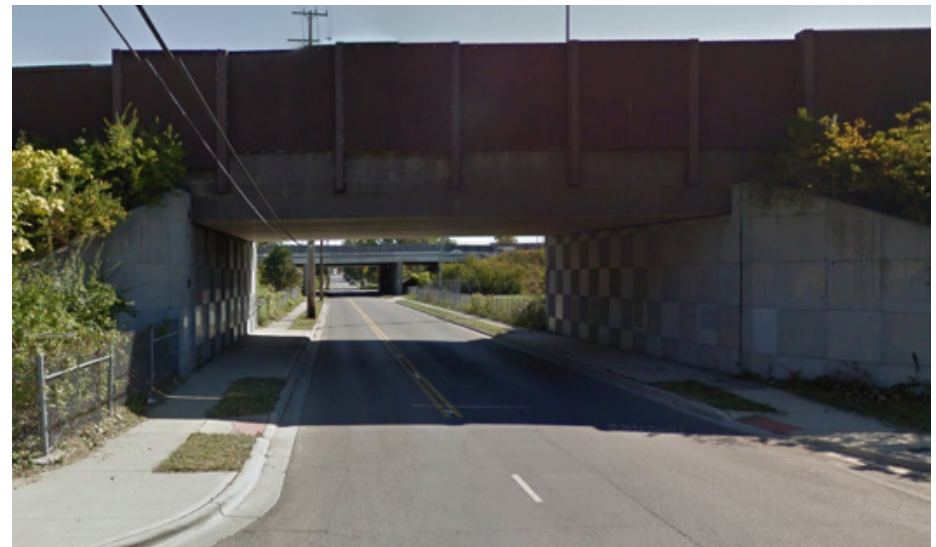
Figure 14: Underpass at 2nd Ave & Washington Ave
